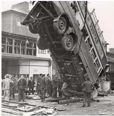
RECOVERY: The effort to rebuild Balham gets underway
