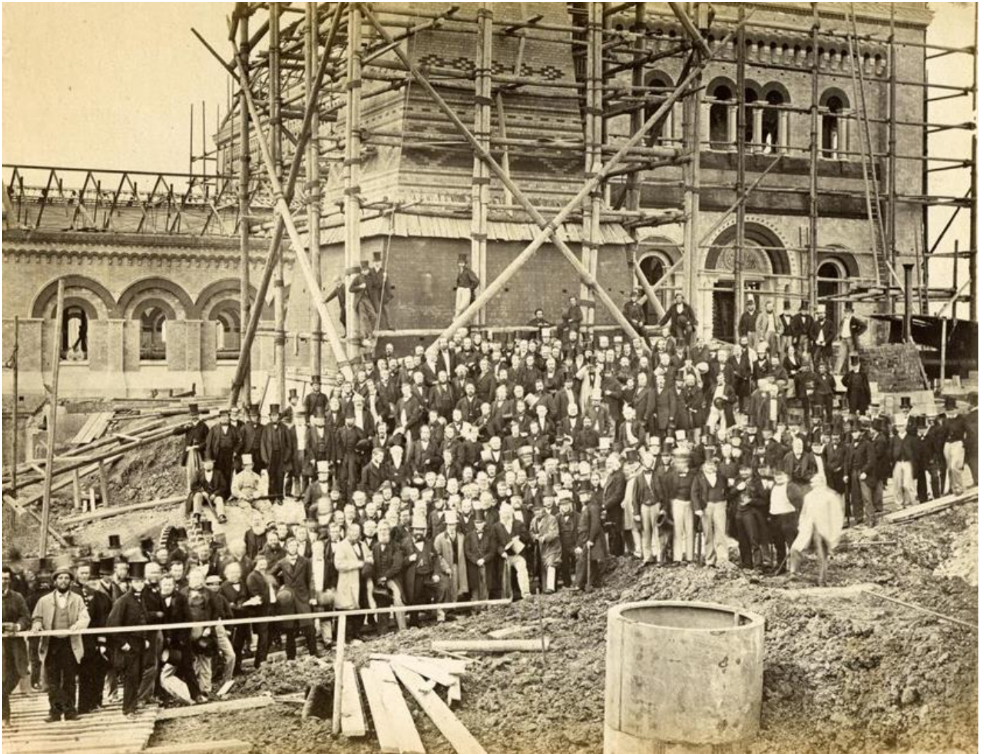
Workmen and engineers at one of Bazalgette's new pumping stations
