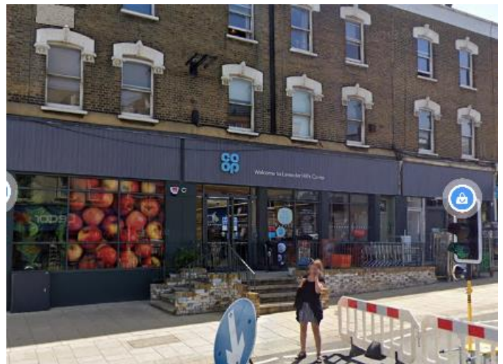
Co-op supermarket Apartments
